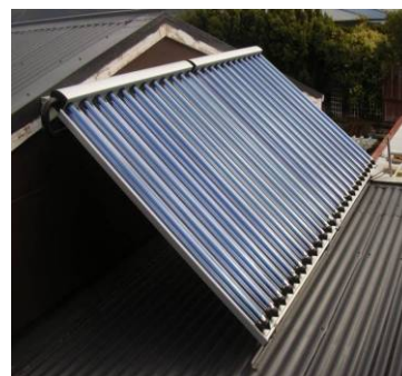
The Papakowhai panels sat at 41° to match the latitude of the site
