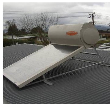
The Rotorua NOW Home panel was limited to 30° by the framing that it came with. It should have been at 38°
