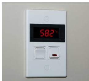
This display in the Waitakere NOW Home showed the homeowners exactly what temperature their solar system was providing
