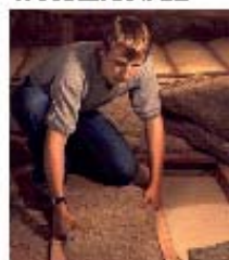
Figure 2 - Installing wool fibre bats
