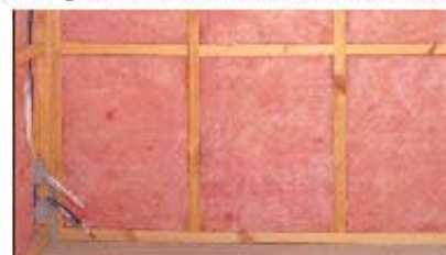
Figure 1 - Glass fibre batts installed in a wall cavity
