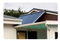
The study also established that solar hot water systems can provide the majority of water heating needs and optimum installations will clearly deliver the best results. The sun's free energy provided an impressive 55-70% of the hot water needs to the three homes with solar water installations – in winter! Summer performance would naturally drive that figure closer to 100%.
